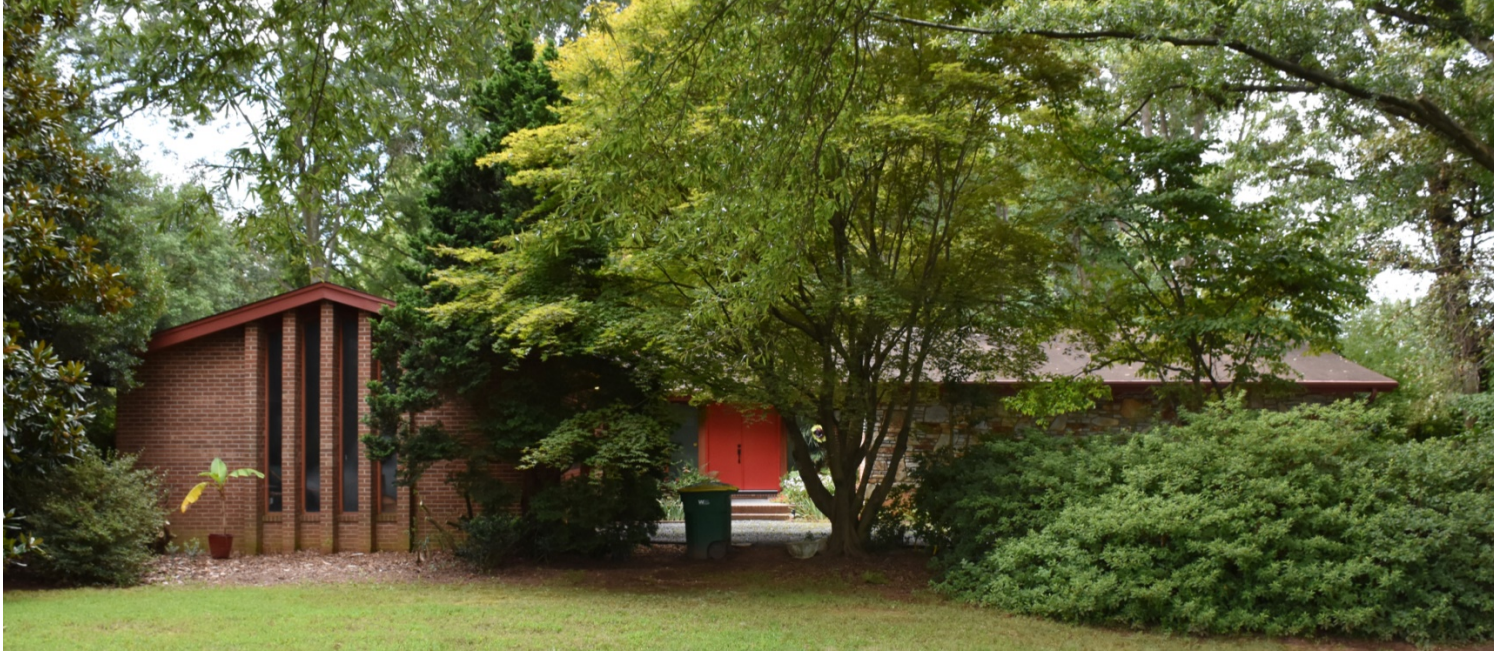
Hank and Georgia Oosthoek House, north elevation
