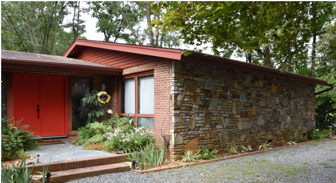
North elevation, west section
